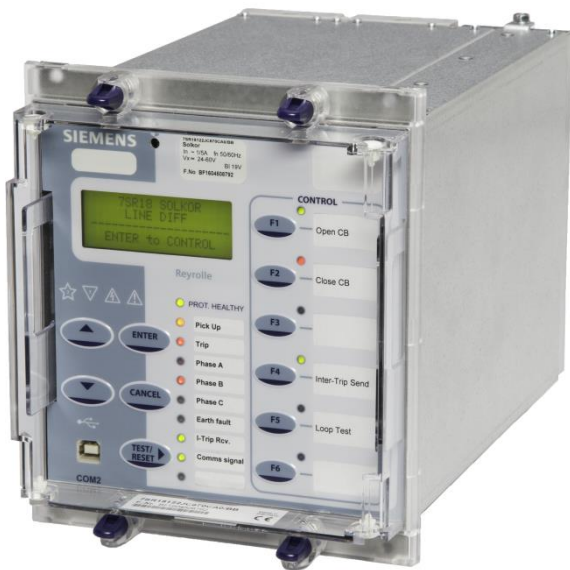
Fig1. Typical Fascia showing additional LED variant
